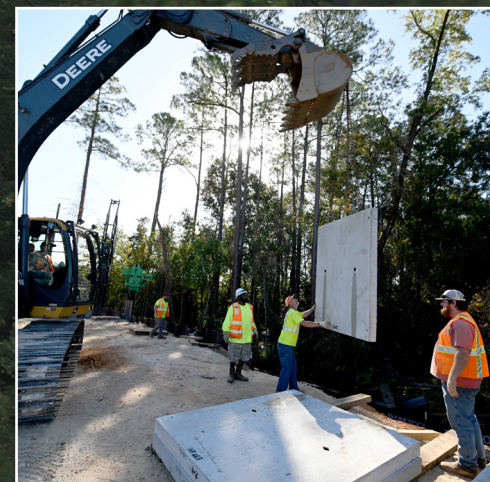
Live Oak Church Road Improvements (In Progress)
