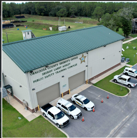
Sheriff's Office Training Center (Complete)
