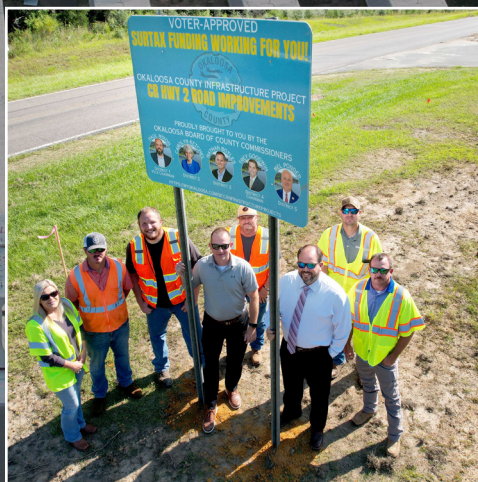
County Road 2 Improvements (In Progress)
